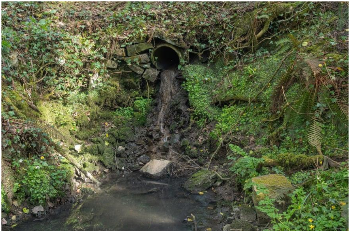
Raw sewage escaping into a river in Carmarthenshire in Wales.
