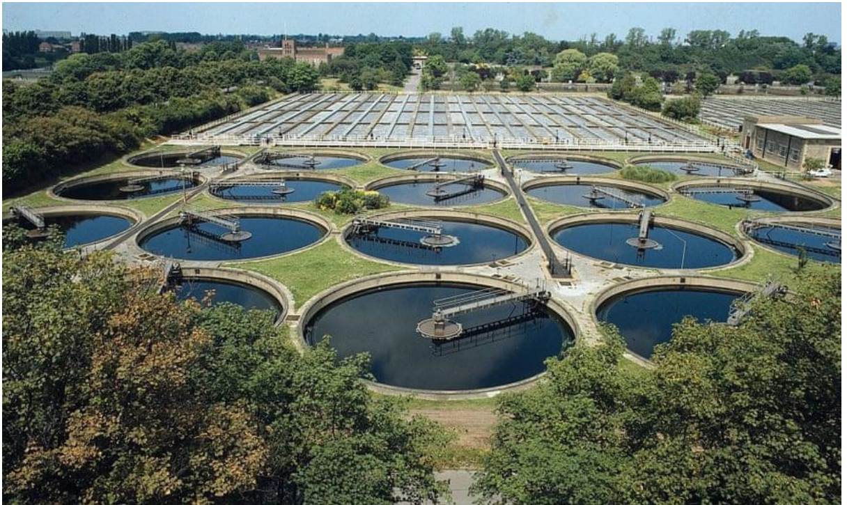
Mogden sewage treatment works in west London.
