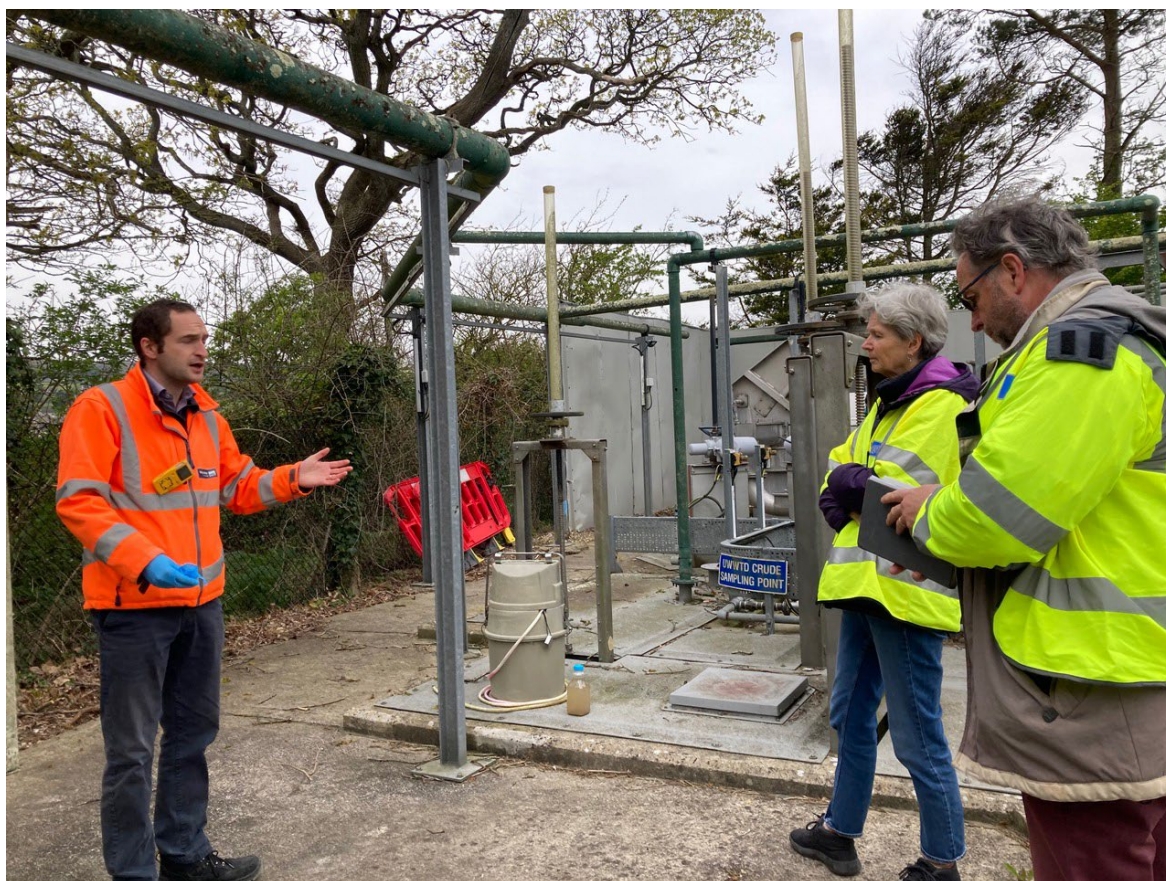
Harry Walker explains how Charmouth's Sewage Treatment Works works
